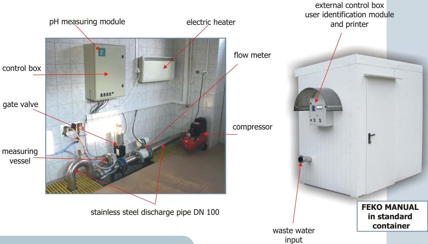
**Sludge water removing system**
